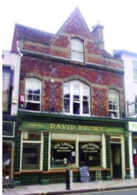
Fig 8: The fascia is the correct depth for the shopfront and the lettering sits well within the frame. The colour scheme is subtle and unifies the whole front - including the door. The stallriser is an appropriate depth.
