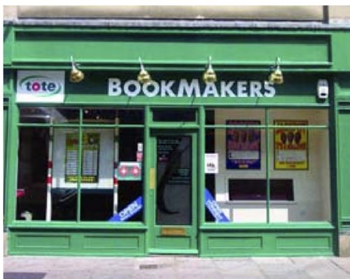
Fig 16: A traditional shopfront with the windowpane divided by glazing bars. The effect is spoilt by the addition of large swan neck lights.
