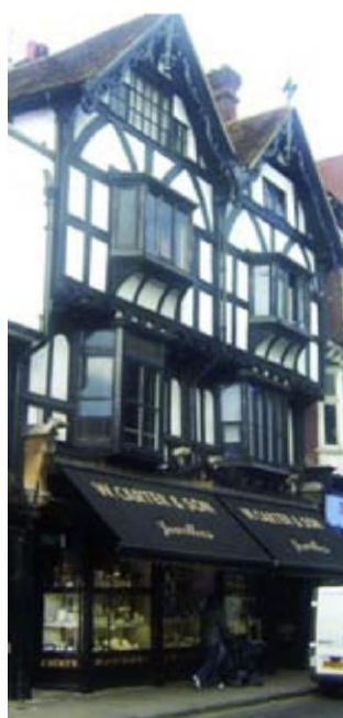
Fig 20: A traditional retractable blind that reflects the character of the shop and does not detract from the upper stories of the building. Because the fascia is covered when it is open, the business name is printed on the blind.
