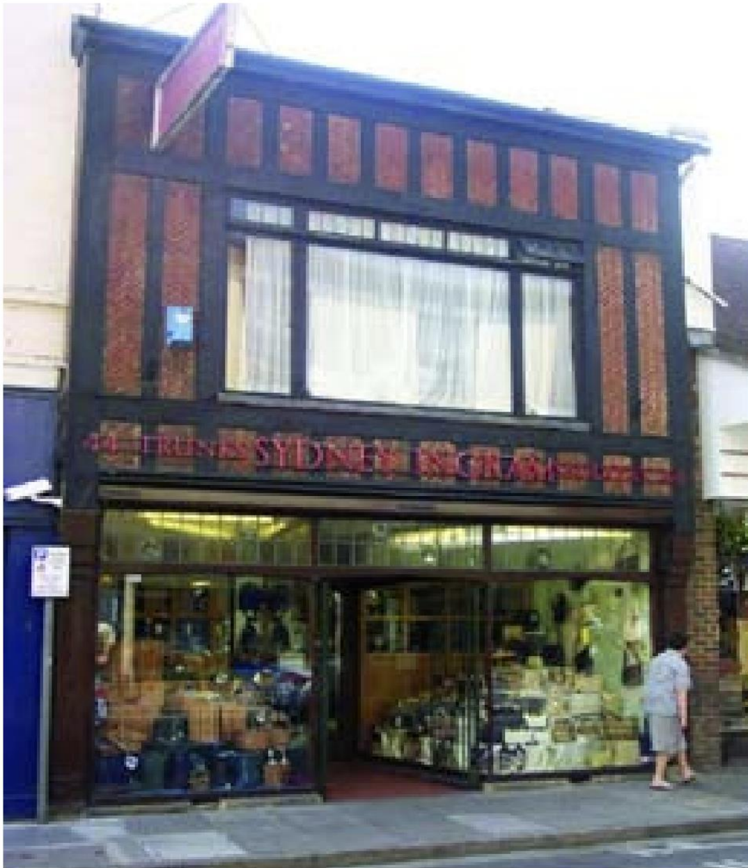
Fig 4: Another example of a recessed doorway. The glass of the shopfront is divided by the Arts and Crafts style leaded lights, which also reflect the style of the building above. There is no fascia so the lettering is applied directly to the building in the fascia position.
