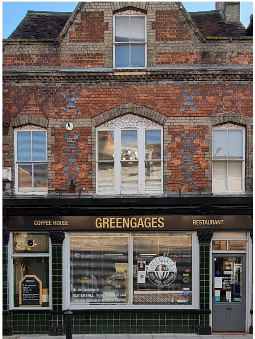
Figure 7: The fascia is the correct depth for the shopfront and the lettering sits well within the frame. The colour scheme is subtle and unified the whole front - including the door. The stallriser is an appropriate depth.
