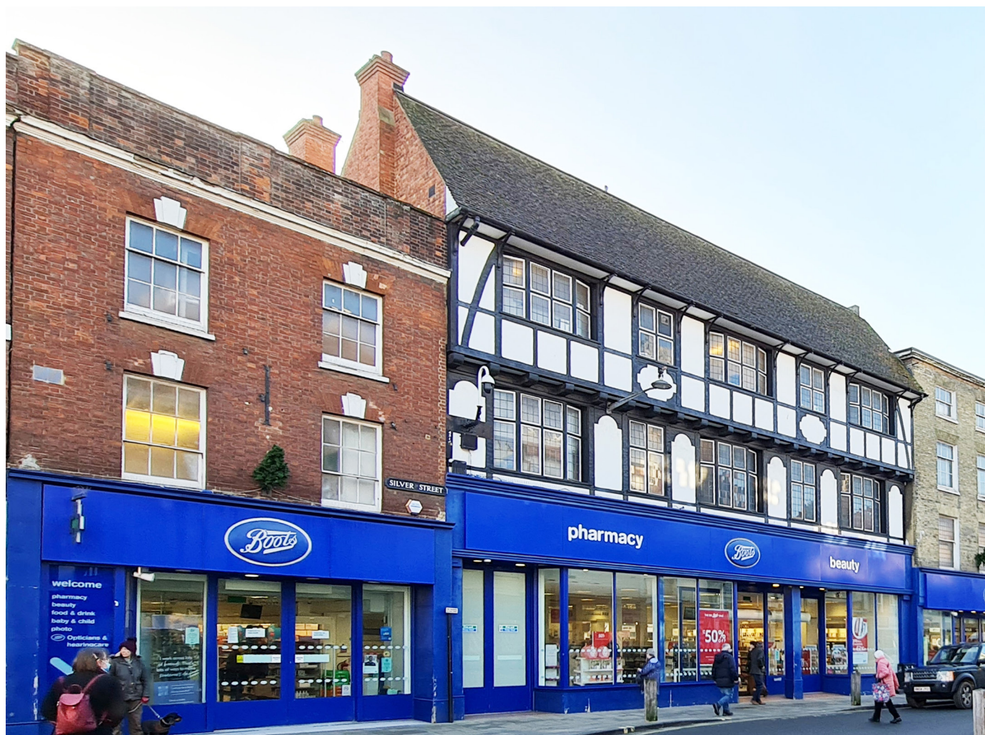
Figure 10: A shopfront with a wide expanse of flat glass. The fascia is made of modern materials and is overly large, impinging on the first floor. The shopfront does not reflect the architecture and the rhythm of the upper floors. The fascia is overbearing and the colouring garish.
