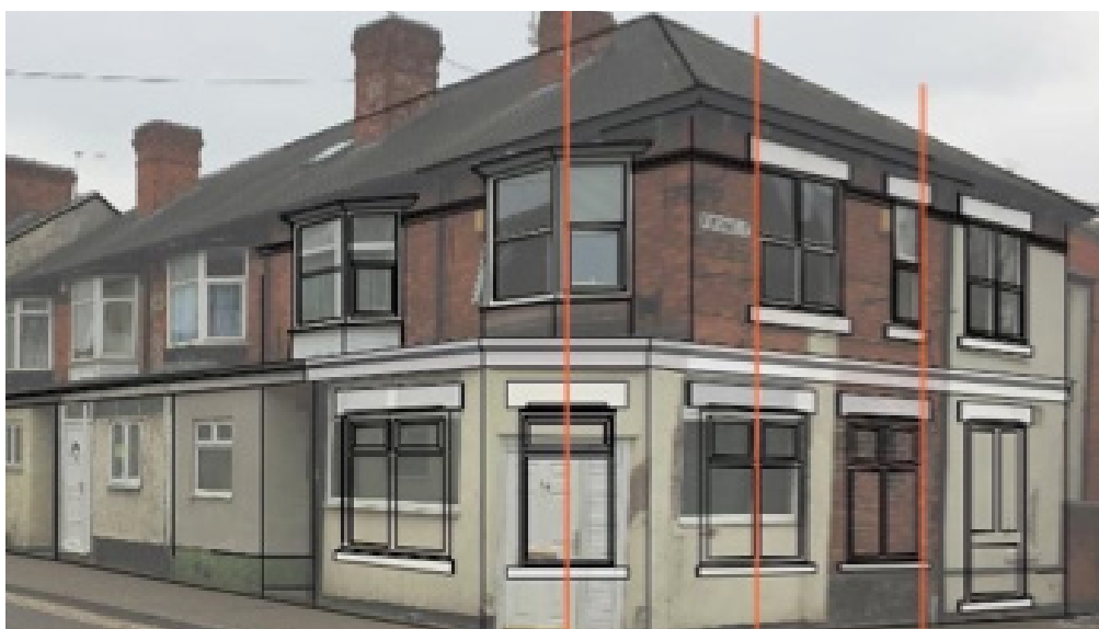
Preferred arrangement. Lower-floor windows are aligned with the upper floor and window heads are replicated.
