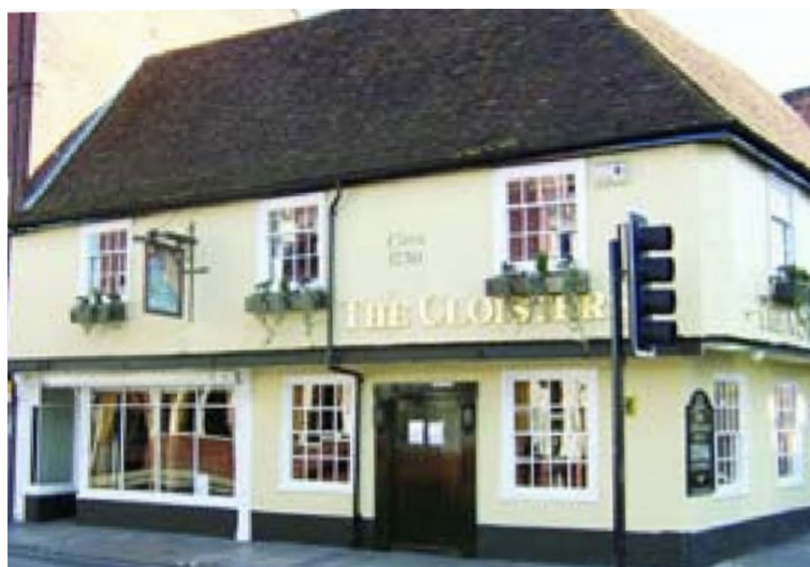
Figure 15: Spotlights are painted the colour of the wall and highlight the signage without being obtrusive
