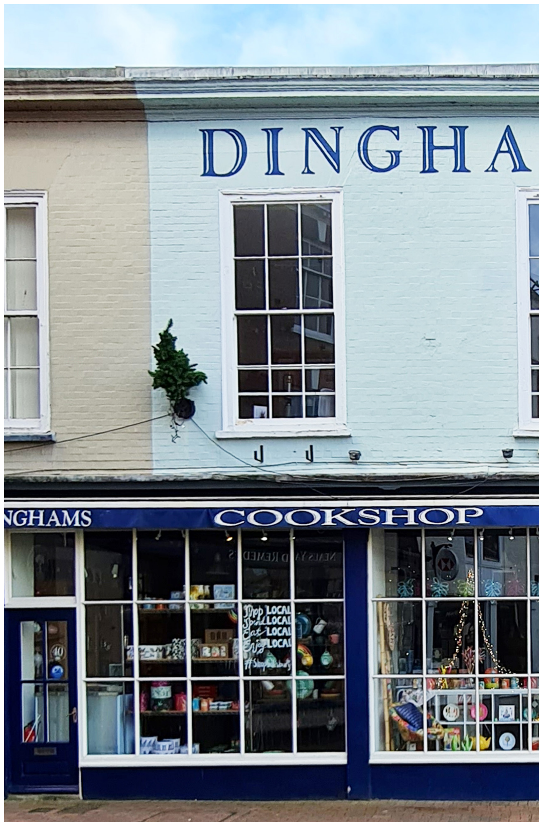
Figure 9: Two potentially large windows are broken up by the glazing bars. These also echo the glazing patterns of the upper floors. Note the painted lettering applied directly to the building at second storey level.
