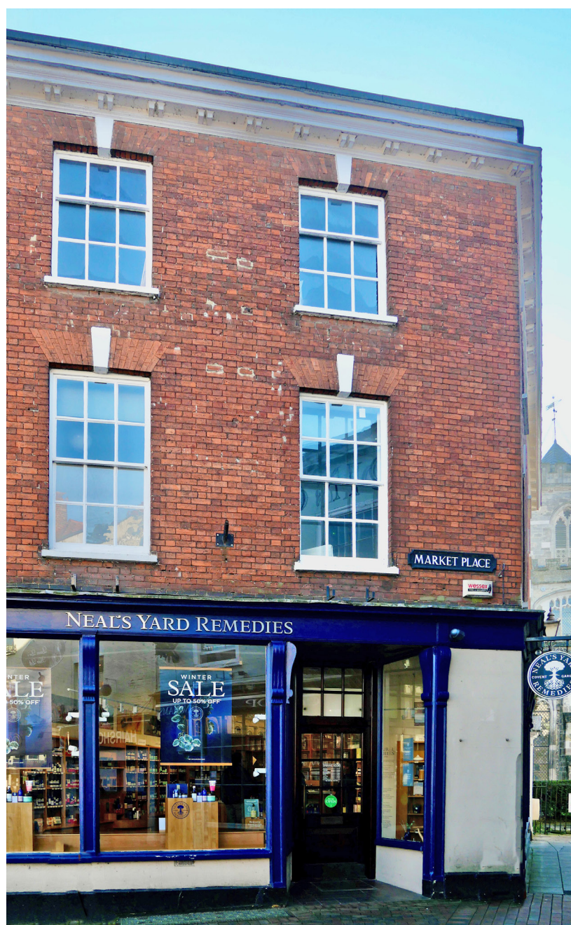
Figure 8: A traditional shopfront utilising a traditional and subtle colour palette. The large glass timber framed window is divided by a mullion.
