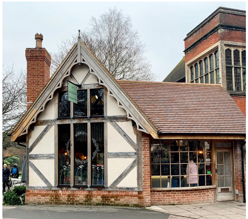
Figure 5: A superb example of a conversion/restoration of a retail shop to a cafe/restaurant (Orangery, Crane Street)
