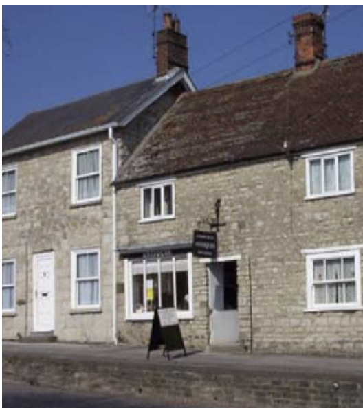
Figure 4: An attractive shopfront in a mainly residential area.
