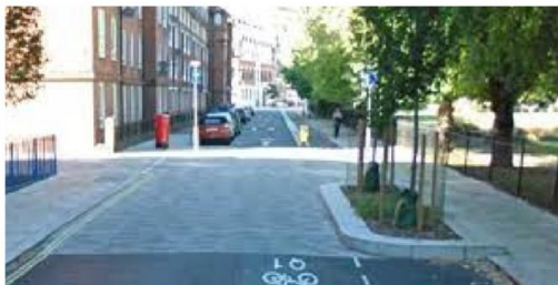
Figure 47. An example of a roadside rainwater garden and a kerbed build-out with tree pits
