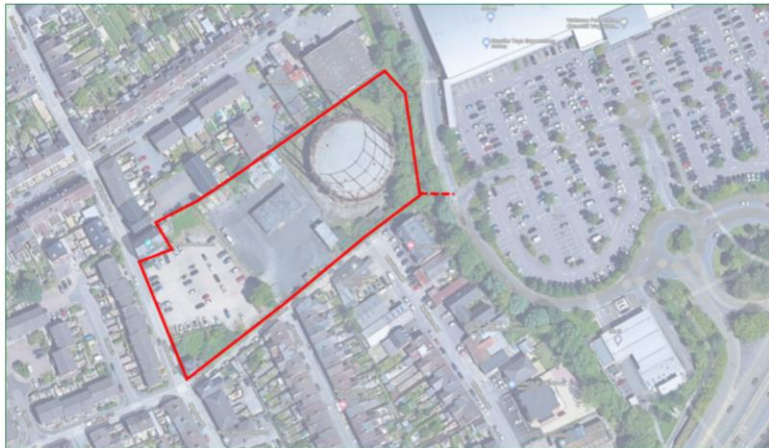
Figure 48. The Coldharbour Lane site showing the gas holder which has now been removed.
