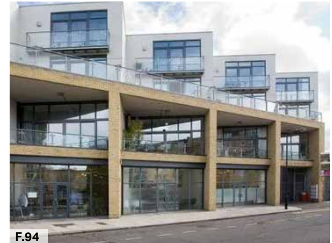
Figure 94: Active frontages with an employment use at ground floor with residential above, Northside studios, source: proplis .
