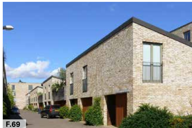
Figure 69: Shared surface with limited car parking along mews street.
