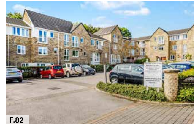
Figure 82: Well overlooked parking court
