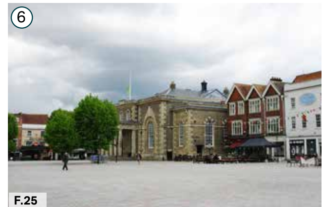
Figure 25: The Guildhall, Grade II* Listed Building.
