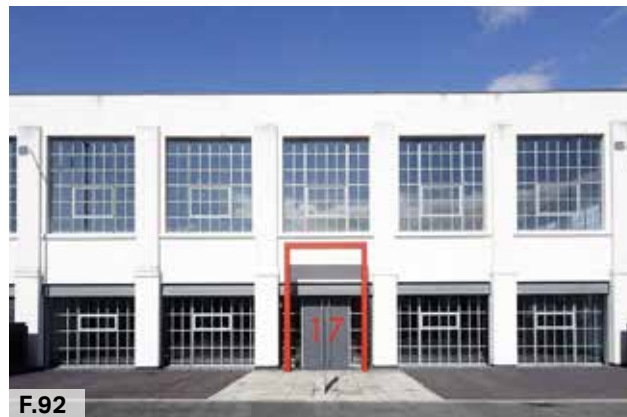
Figure 92: Stacked medium and small employment units, Matchwork Studios, Liverpool, Source: Place North West
