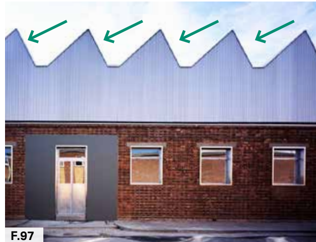
Figure 97: Light from the roof reduces the need for windows on the top floor, Sackler Building, Source: Helene Binet.
