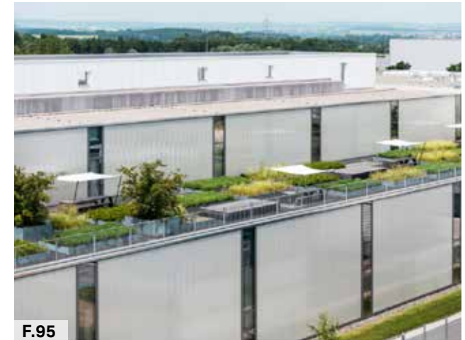
Figure 95: Uhlmann factory with a roof terrace, source: Barkow & Leibinger Architects .
