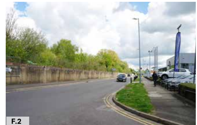
Figure 02: View along Lower Road with the Engine Shed site to the left and the Churchfields Industrial Estate to the right.
