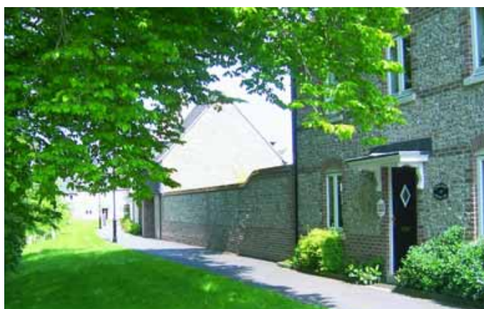
Above This new property shows good flint detailing, where the material is used in a generous way in a proportion with the brickwork that reflects the traditional pattern. There can be a modern tendency to insert flint to try and reflect the local character, but in a rather mean cursory way which only leads to a cheap parody of the original building style.
