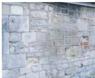
Above The use of ribbon pointing that stands proud of the stonework is inappropriate, uncharacteristic of the area and spoils an otherwise fine wall
