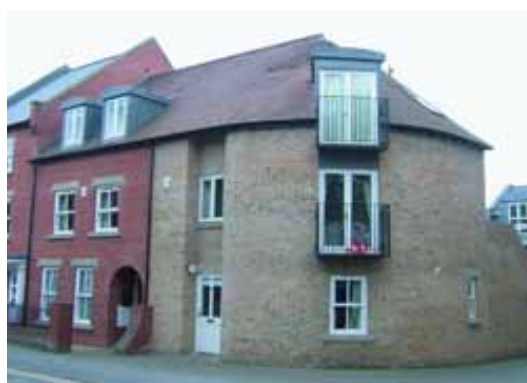
Above High quality contemporary infill on the street frontage in Salisbury, which respects historic patterns of development and harmonises well with the existing town
