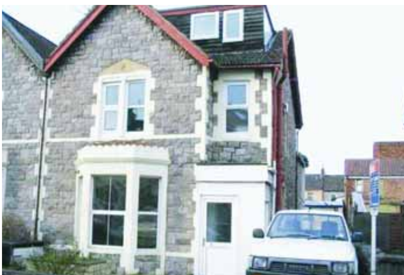
175 The dormer on this traditional stone Victorian villa is especially crude and ruins the architectural quality of the original fine property
