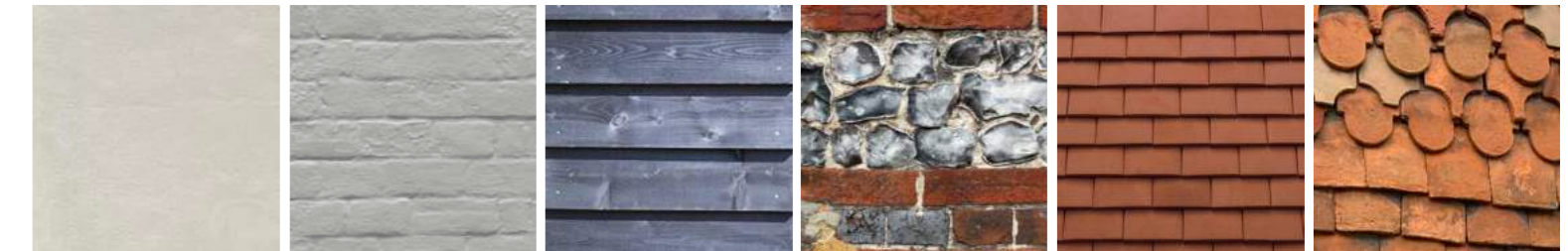
Variations in wall finish, painted brick, painted render, hung clay tiles, stained timber cladding and knapped flint courses
