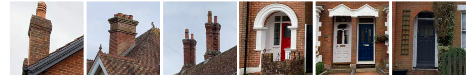
Other notable features: chimneys, recessed porches, deep hood moulds to windows
