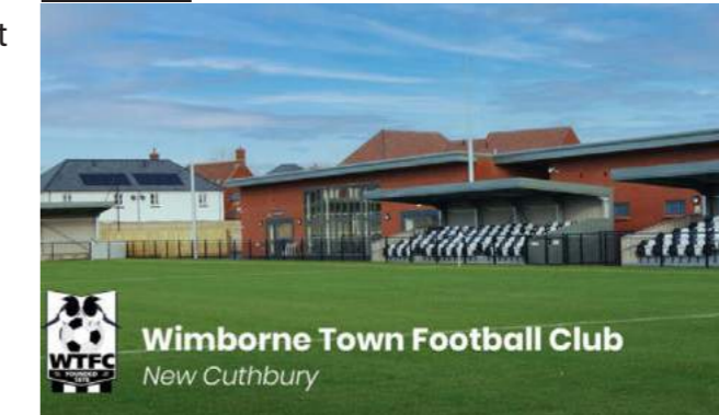
New football club ground and facilities for Wimborne
