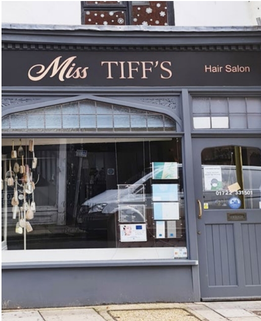
Above An attractive glazed shopfront in Catherine Street.
