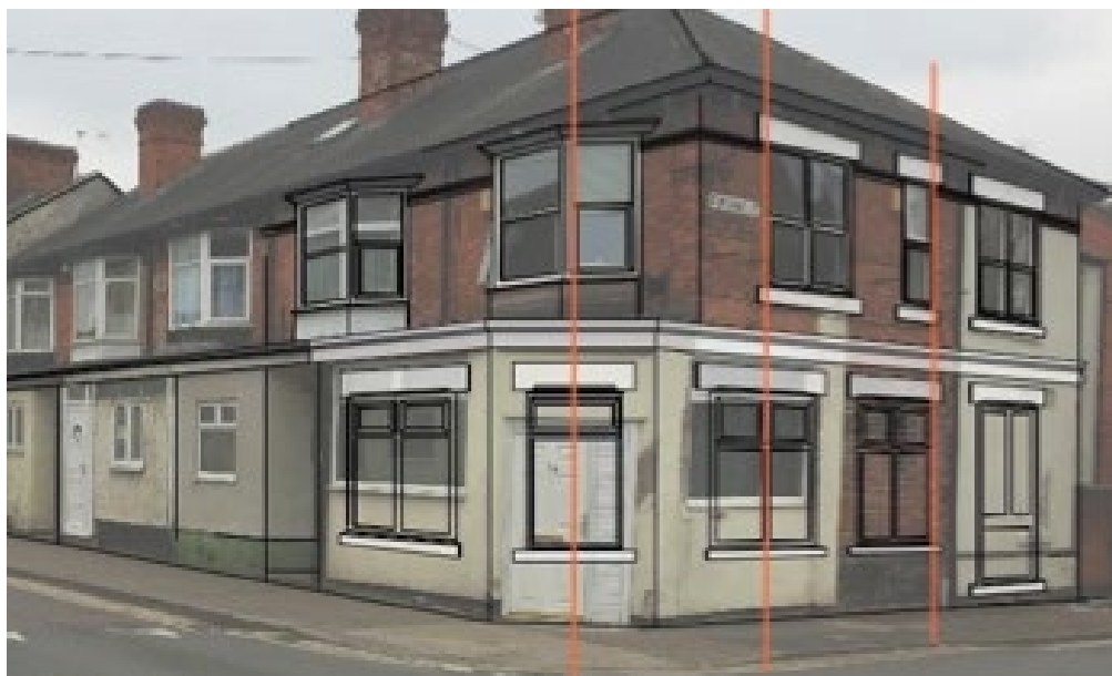
Preferred arrangement. Lower-floor windows are aligned with the upper floor and window heads are replicated.
