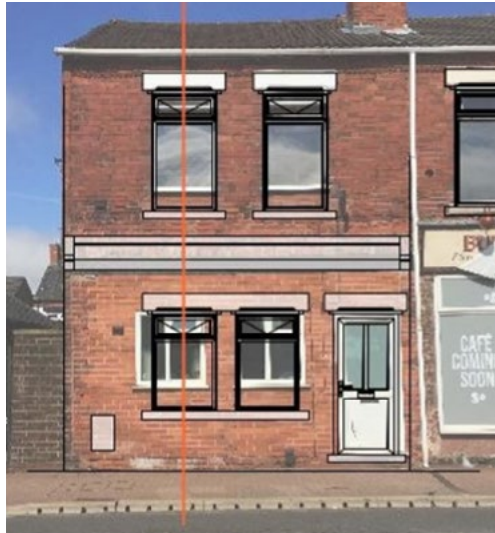
Preferred arrangement. Lower-floor windows aligned with upper floor and window heads are replicated.
