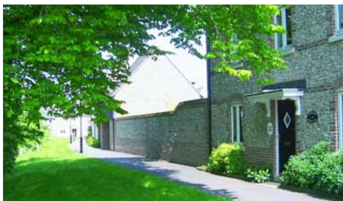
Above This new property shows good flint detailing, where the material is used in a generous way in a proportion with the brickwork that reflects the traditional pattern. There can be a modern tendency to insert flint to try and reflect the local character, but in a rather mean cursory way which only leads to a cheap parody of the original building style.
