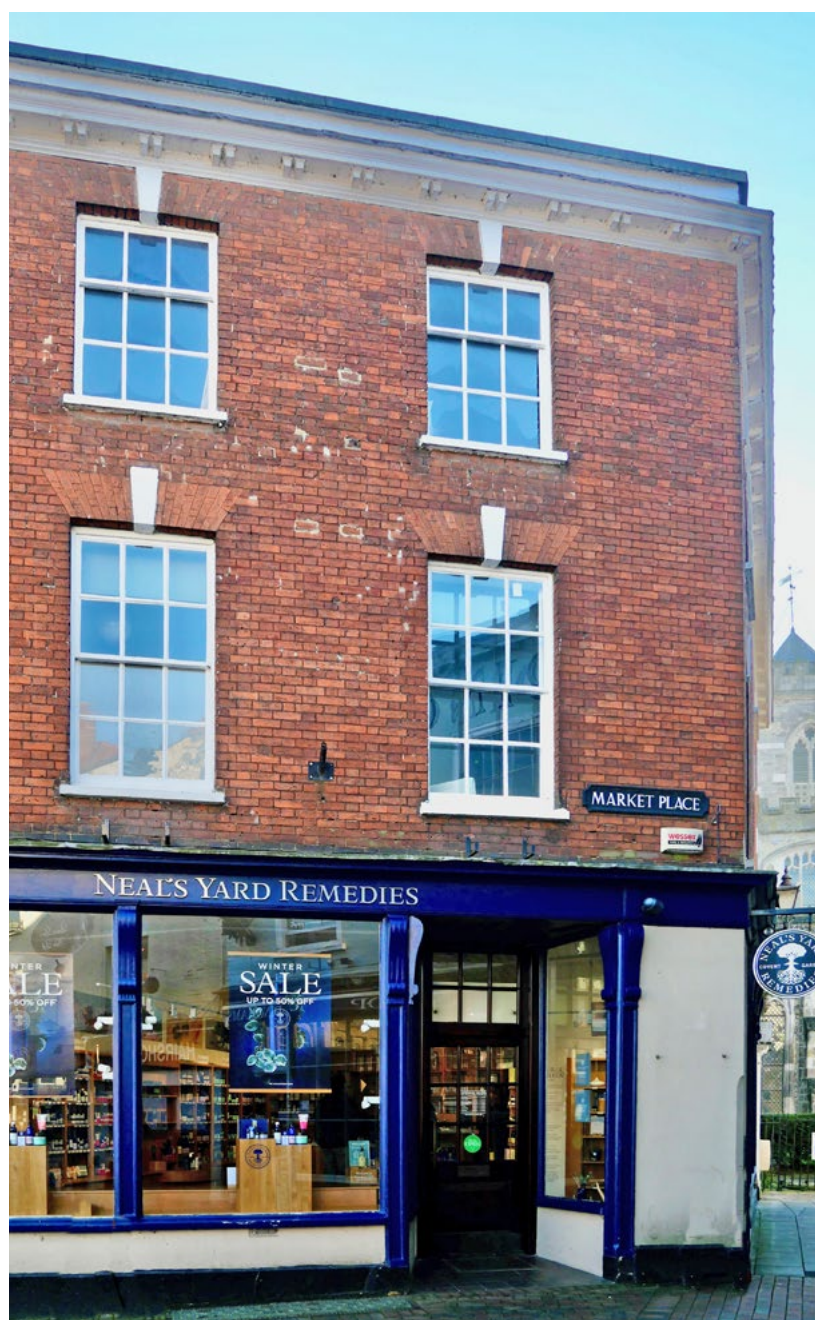
Above A traditional shopfront utilising a traditional and subtle colour palette. The large glass timber framed window is divided by a mullion.
