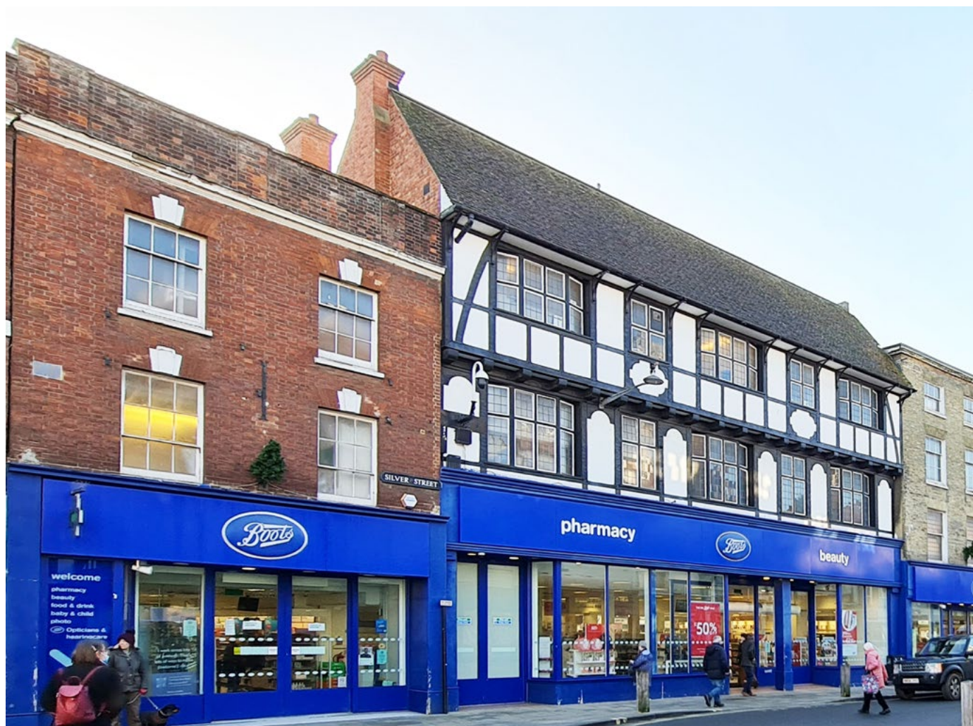
Above A shopfront with a wide expanse of flat glass. The fascia is made of modern materials and is overly large, impinging on the first floor. The shopfront does not reflect the architecture and the rhythm of the upper floors. The fascia is overbearing and the colouring garish.
