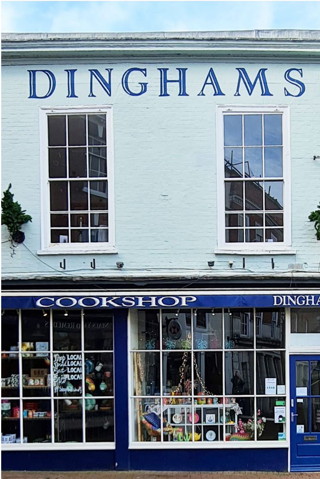
Above Two potentially large windows are broken up by the glazing bars. These also echo the glazing patterns of the upper floors. Note the painted lettering applied directly to the building at second storey level.
