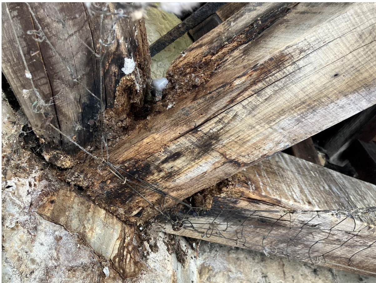
Fig 9: Poultry Cross, 2025: High level inspection of internal roof structure; significant decay at beam ends and junctions in timber structure.
