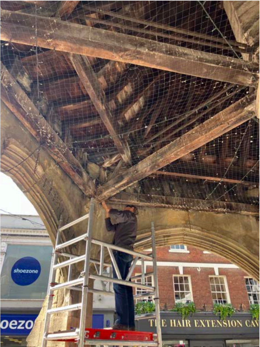
Water ingress to majority timber and boards
