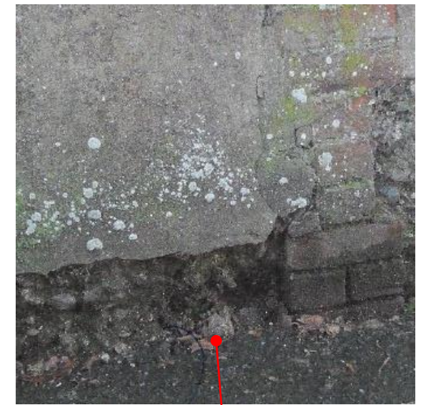
Loss of wall material at base.
