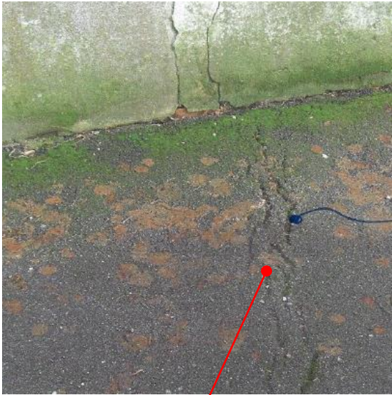
Damage to the footpath from tree roots.
