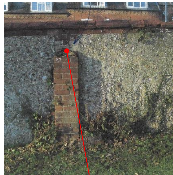
Top of pier is missing and weathering of the wall.
