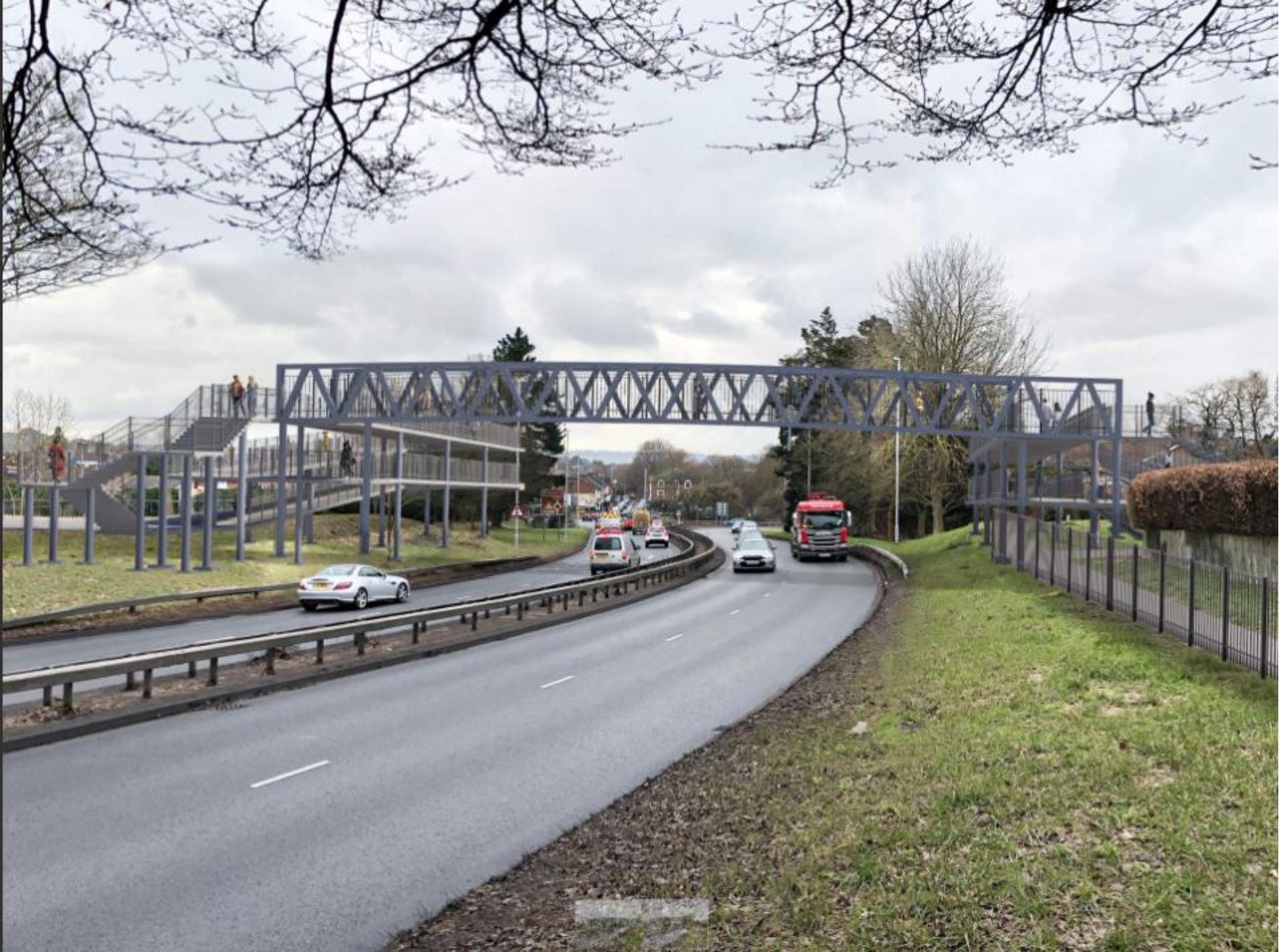
Victoria Road Replacement Footbridge
