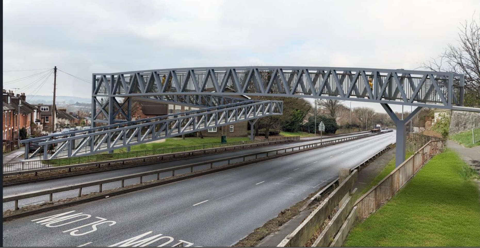
Wyndham Road Replacement Footbridge
